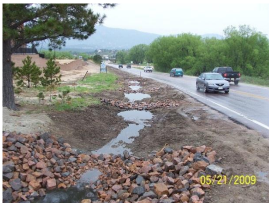
Excellent installation of rock check dams.
