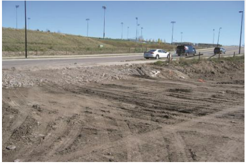
Poor installation of a Vehicle Tracking Pad. It is not 70 feet long. Refer to the table below for details.
