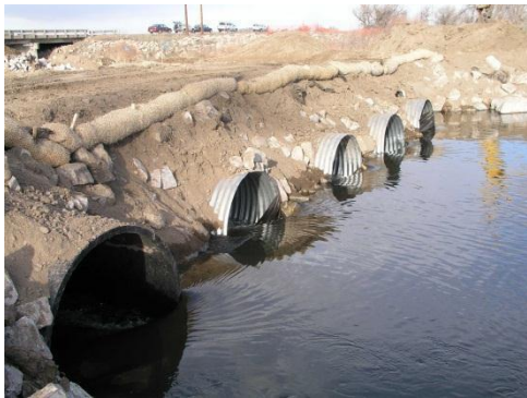
No riprap at approach to prevent sediment from entering the stream.
