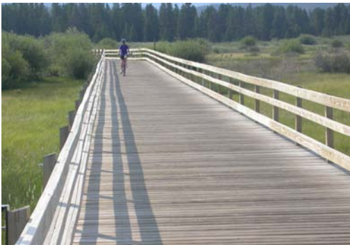
Example of Deck Near Frisco
